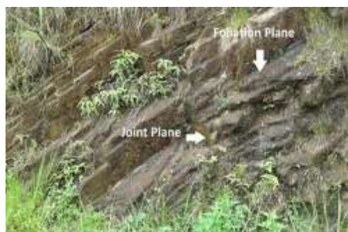
Fig. 1. An image showing rock outcrop with strongly developed major geological discontinuity planes such as foliation and joints planes. Location - road cut along Balangoda- Haputale road.
